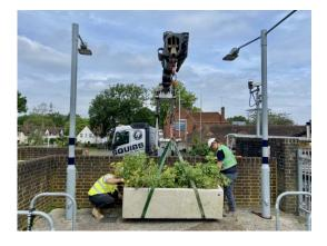
The high reach excavator, which recently arrived on site, commenced enabling works on Friday. These works are to facilitate the relocation of another machine, so that the demolition can commence on schedule on Monday 12 July.
